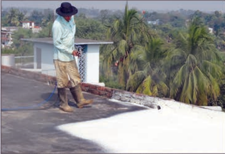
PUF Spray on Roof top of Cold storage
