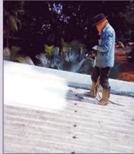
PUF Spray on Asbestos Roof sheet
